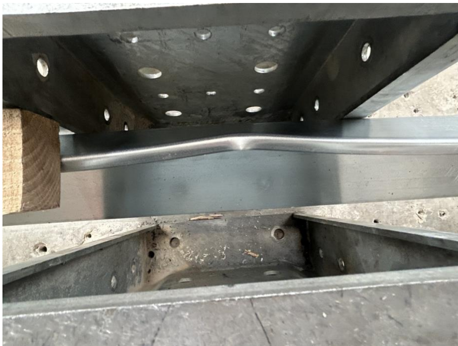
Figure 6 – Z Perlin Failure
