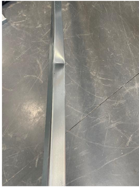
Figure 3 – C Purlin Failure
