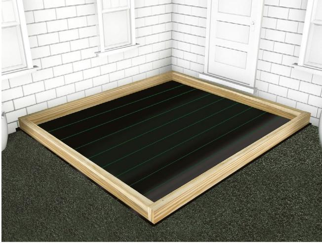
**1** Prepare a level, weed-free area for the deck. To create a framework, cut the joists (using either a 47mm x 100mm or 47mm x 150mm) to the required length, then join using exterior wood screws. Check the frame is square, by measuring diagonally from corner to corner. If installing on grass or soil, use a weed mat to ensure weeds do not grow through from the base of the Decking frame.
