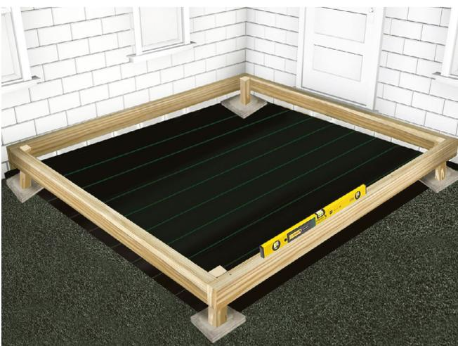
**3** If your deck will be sitting on grass or soil, you will need to place blocks or slabs underneath each leg, to spread the load and provide a level, stable base. Additional blocks can be used if required. Position and adjust the blocks/slabs, ensuring the frame is at a slight angle, that will allow the water to drain down the length. We recommend a slope of at least 5mm for every metre. Alternatively, if using slabs, you could dig a hole and set the legs in concrete.
