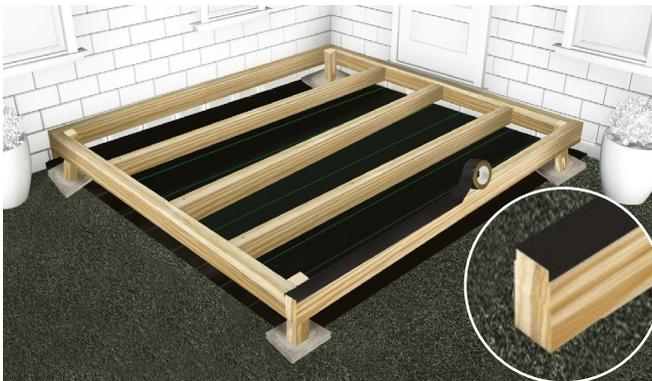
**5** Measure across the inside of the frame at your joist marks, then cut lengths of (47mm x 100mm) or 47mm x 150mm) timber to suit. To fix the joists, tap them in with a hammer until flush with the top, ensuring they do not push the frame out of shape. Then screw them in place from the outside of the frame. Apply Deck Tape to the top surface and cut ends of joists to protect them from moisture.
