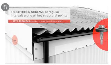
Stitcher screws are recommended to secure flashings. Screws should be no more than 400mm apart when securing the flashing. Colour caps can be used to conseal the top of the screw head.
