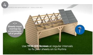
When installing the box profile sheeting you may wish to lay the sheets on the roof before fixing to ensure the overlap is sufficient. Sheets should be overlapped by a minimum of one tile profile when laid side by side.
