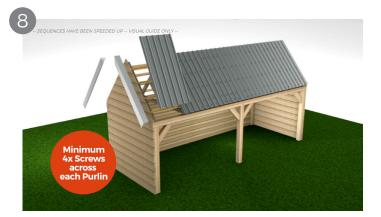
Once you have installed the final sheet you can use Cladco flashings for the sides and apex. Barges are used on the edges to help seal the building and provide an aesthetically pleasing affect. Please note when joining / laying these there is a minimum overlap of 200mm on barges. Our 22mm stitcher screws are advised for securing flashings in place.
